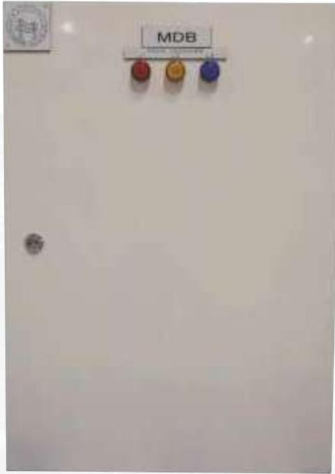
Main Distribution panels are cabinets that house and separate subsidiary/branch circuits in addition to providing each circuit with protective fuses or circuit breakers.
